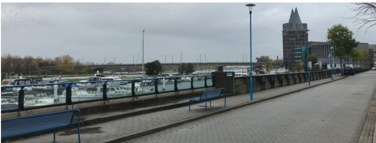
Glazen waterkering in Roermond
