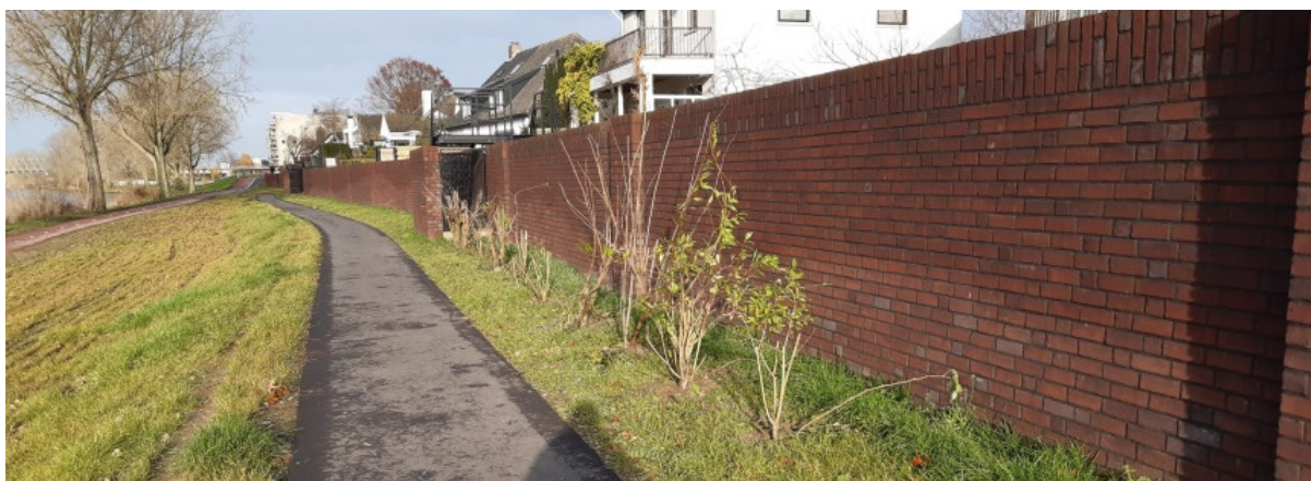
Harde waterkering in Mook
